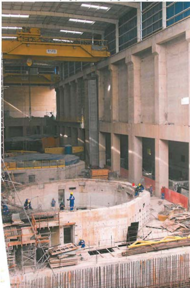
Picture 11. Powerhouse interior facing left wall – Unit 2 in foreground (January 6, 2014)
