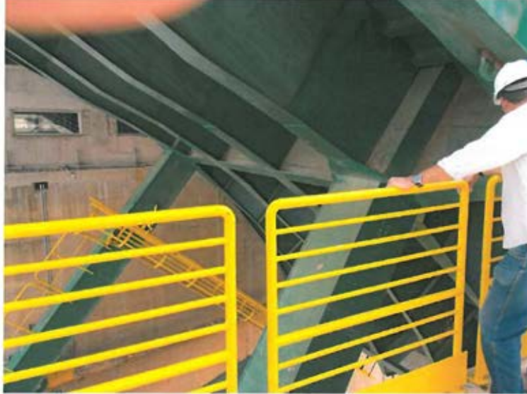
Picture 18 – Downstream Face of the Three Spillway Gates in Opened Position (January 6, 2014)
