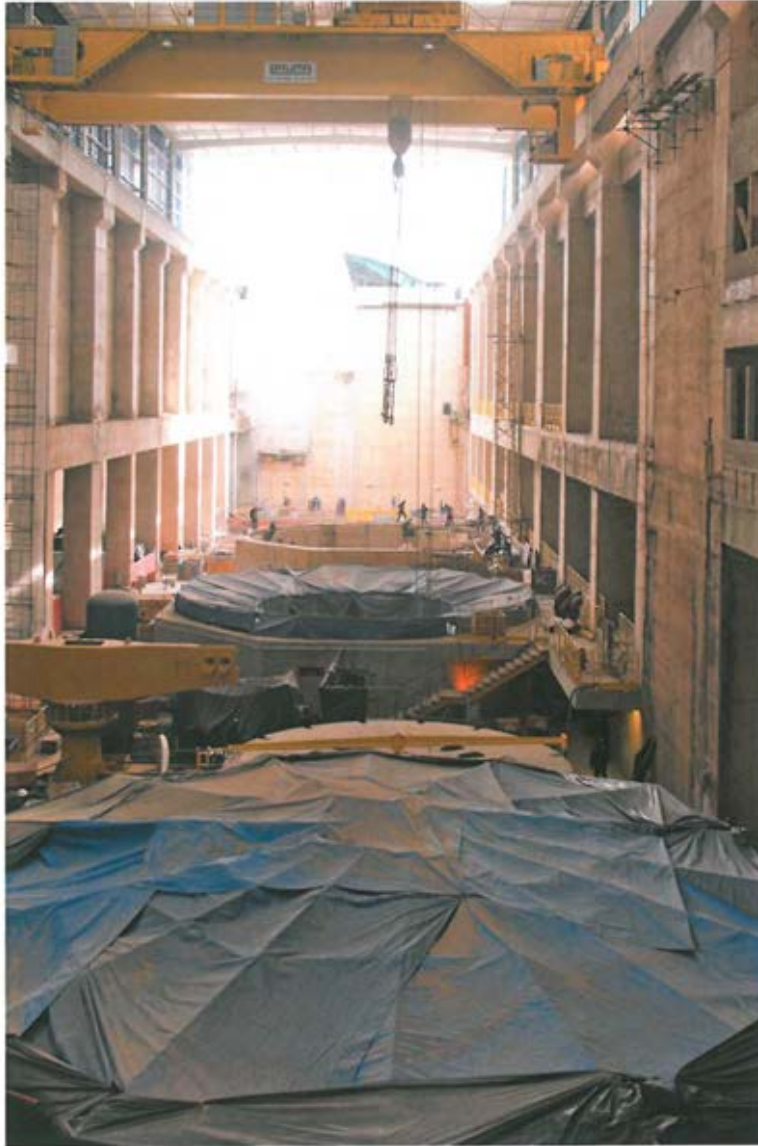
Picture 12 Powerhouse interior facing right wall (January 6, 2014)
