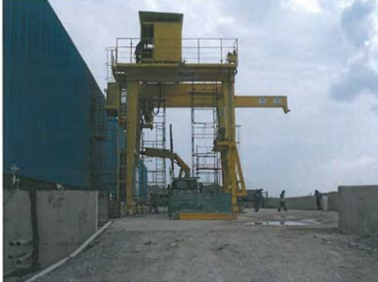
Picture 10. Upstream Wall of Powerhouse and Crane for Operation of Intake Stop-Logs (Jan 6, 2014)
