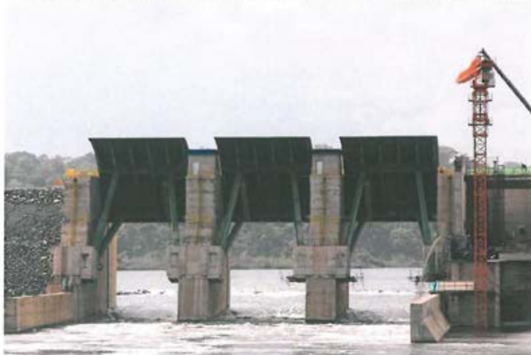
Picture 18 – Downstream Face of the Three Spillway Gates in Opened Position (January 6, 2014)
