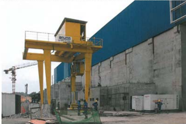
Picture 8 Downstream Wall of Powerhouse and Crane for the Operation of Draft Tube Stop-logs
