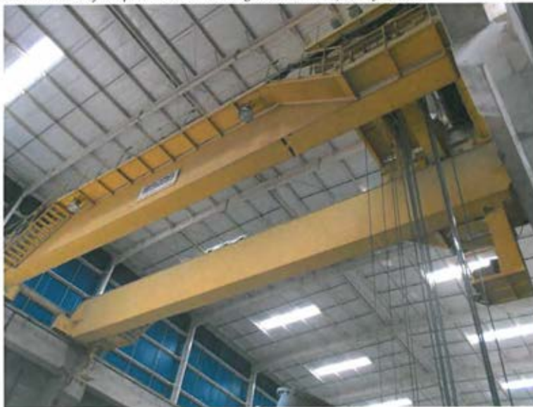
Picture 16. One of two powerhouse cranes being used at Unit 1 (January 6, 2014)
