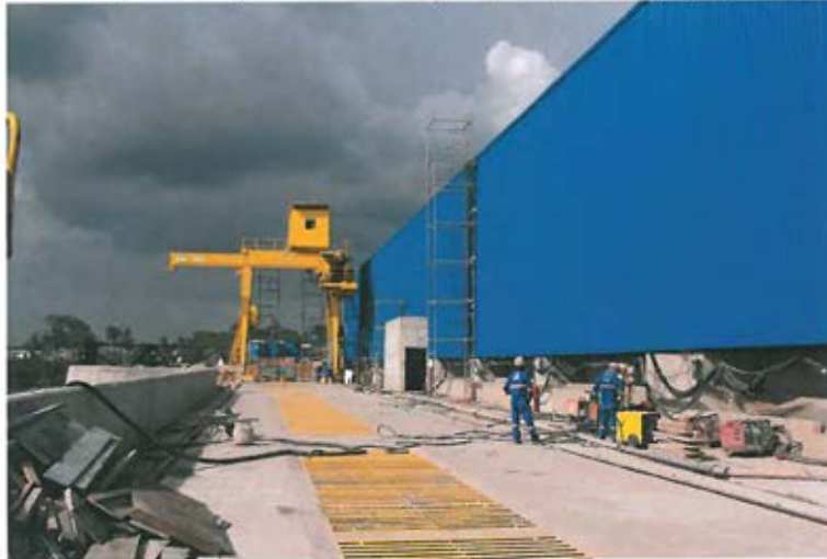
Picture 10. Upstream Wall of Powerhouse and Crane for Operation of Intake Stop-Logs (Jan 6, 2014)
