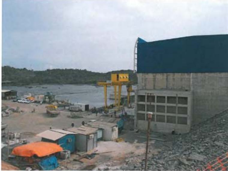
Picture 8 Downstream Wall of Powerhouse and Crane for the Operation of Draft Tube Stop-logs
